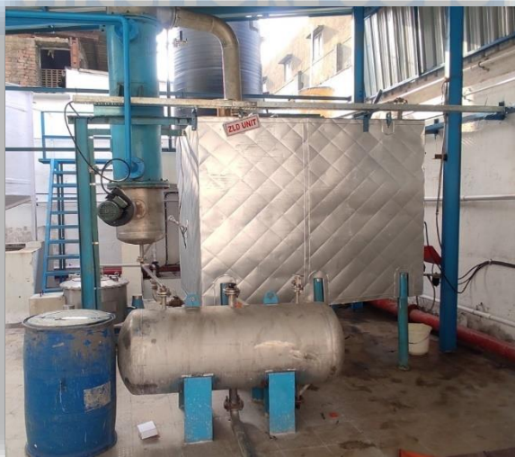
Gas Fired Wastewater Evaporator
